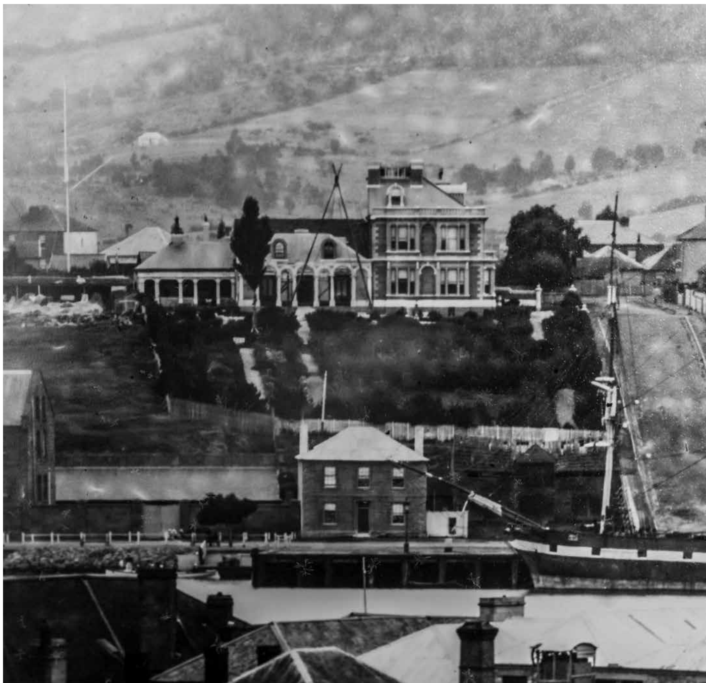
Lenna taking shape in stages; notice the original Bayley House left of the new Lenna.
