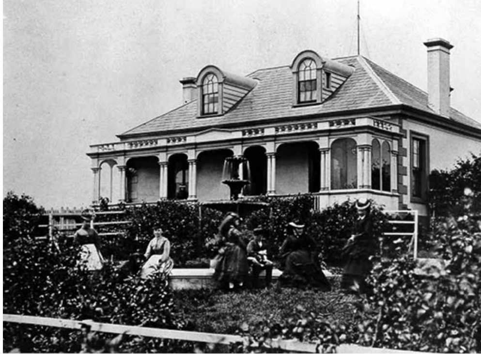
The original Bayley House and fountain; these dormer windows still visible on top of Lenna.
